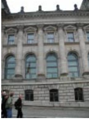
Renovation of a historical facade, Berlin
