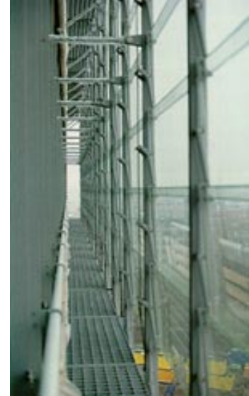
View from within the interstitial space.
