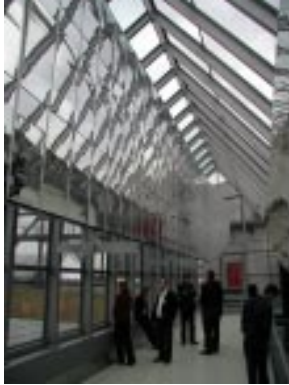
Light-redirecting skylight, Berlin.
