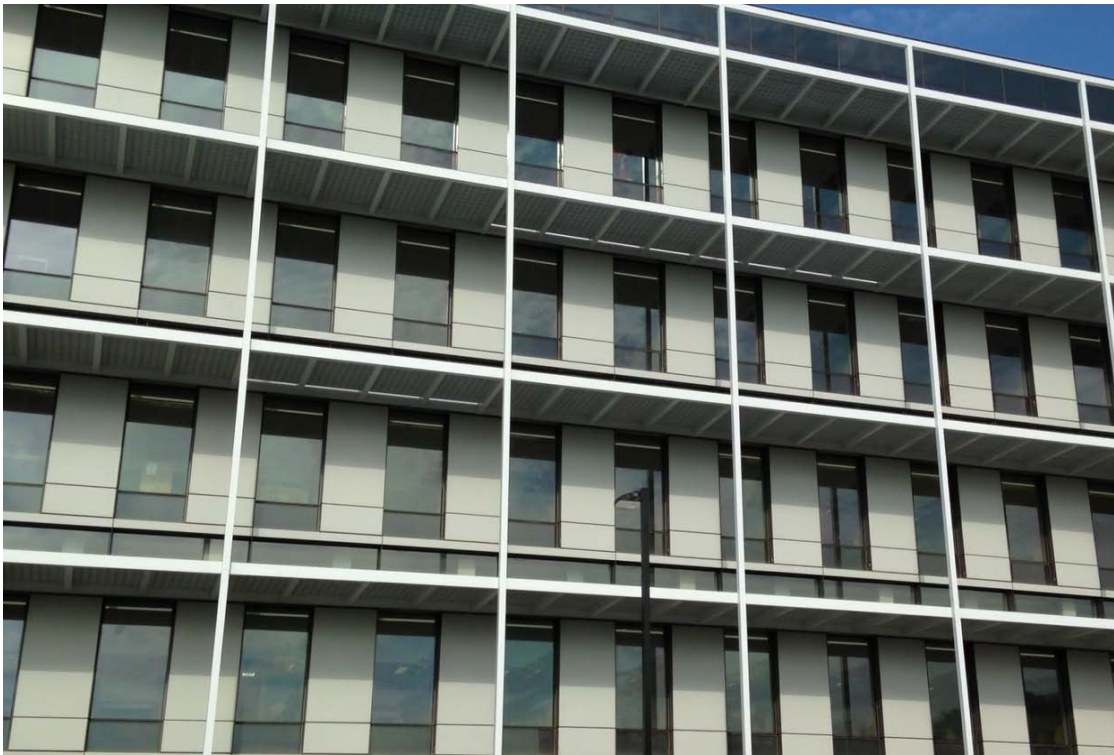
Figure 60: Exterior view of a typical daylit laboratory
