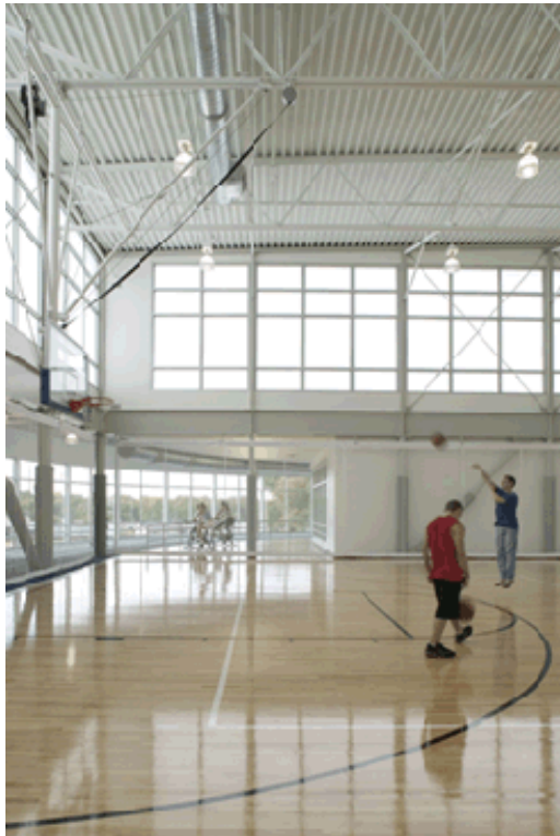
Translucent clerestory panels, Kirkwood Community College Recreation Center, Cedar Rapids, Iowa, Architect: Neumann Monson, Iowa City, Iowa. Photo: Farshid Assassi, Assassi Productions, Santa Barbara, California at www.advancedglazings.com
