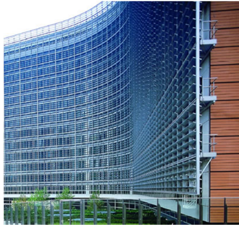
Automated louver systems on the European Commission Headquarters, Berlaymont, Brussels, Belgium. Photo: Colt International Limited.
