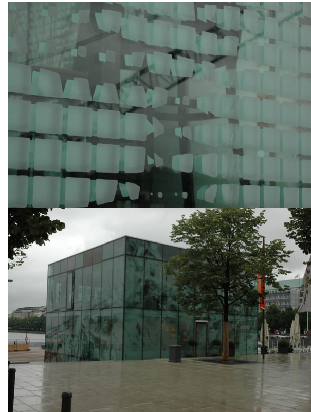
Glass pavilion in Hamburg, Germany. A graphic pattern of frits provides some reduction of solar heat gain. Photo: Mark Perepelitza
