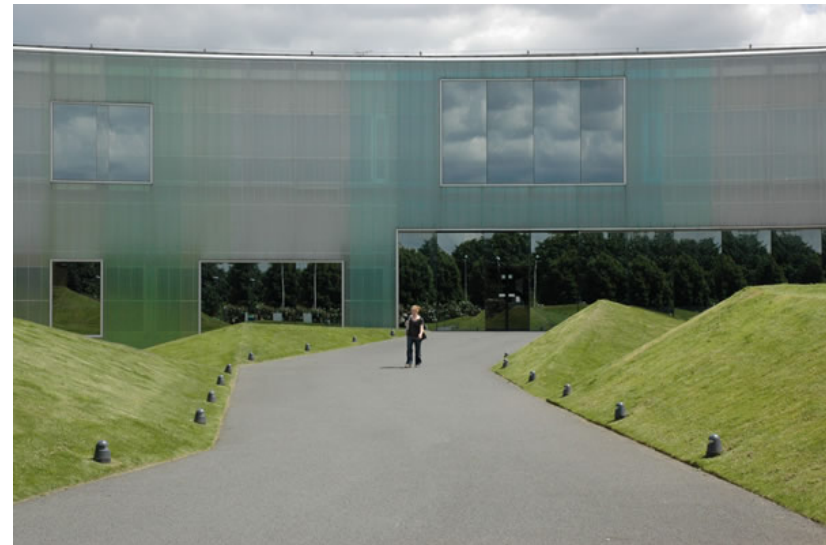
Laban Dance Center, London, UK, Herzog de Meuron Architects. Color tinted translucent polycarbonate is used for the majority of the outer skin with glass windows interspersed. In the dance studios the walls glow during the day, and at night the entire building exterior glows with the color and silhouettes of activity within. Studies of the buildings energy performance and visual comfort have shown mixed results. Photo: Mark Perepelitza
