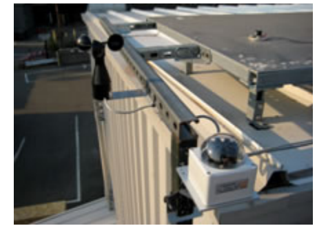
Integrated microprocessor and runtime motor controller in a weatherproof box (left) is used to actuate the blinds (left). Brightness sensor and wind anemometer located on the roof (right). Photo: LBNL.
