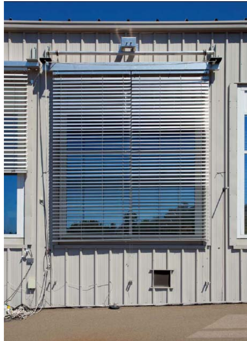
Exterior view of zoned, optical exterior louver system. Photo: LBNL.
