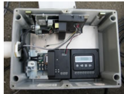
Integrated microprocessor and runtime motor controller in a weatherproof box (left) is used to actuate the blinds (left). Brightness sensor and wind anemometer located on the roof (right). Photo: LBNL.
