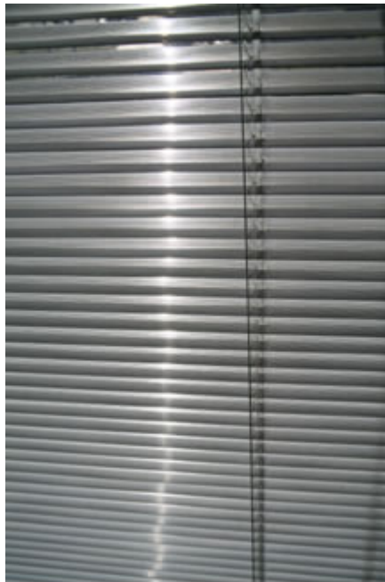
Specular reflections of sunlight off shiny slat surfaces can cause glare discomfort glare.
