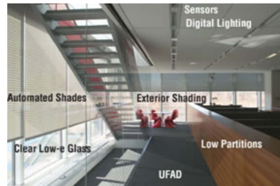
Automated shades and digital lighting controls for The New York Times Headquarters Building. Photo: David Joseph.
