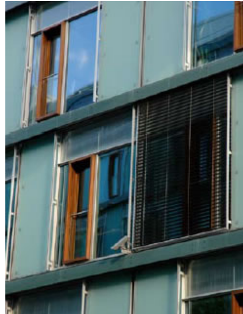
Jakob Kaiser Haus, Berlin Germany, Busmann + Haberer Architects Automated exterior blinds integrated into the façade. Photo: Mark Perepelitza
