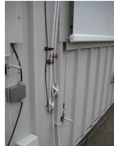
The lower hem bar is restrained by a vertical guide wire that runs the height of the window. Photo: LBNL.
