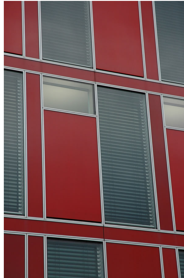
Capricorn Haus, Düsseldorf, Germany, Gatermann Schossig Architects. Continuous daylight glazing, but reduced overall glazing area in a unitized, double-skin facade. Photo: Mark Perepelitza
