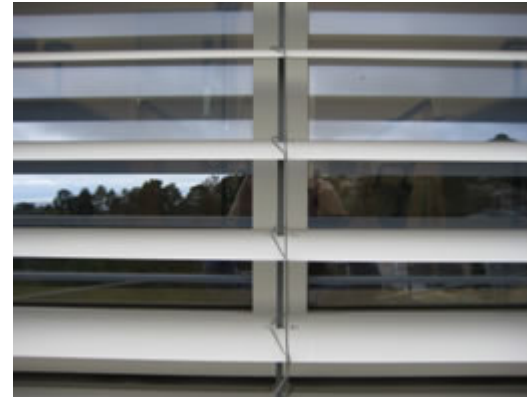
100-mm (3.9-inch) slats with semi-gloss white finish on top and bottom surfaces resting on braided plastic string ladders. Flat Trevira-polyester ribbons are used for lift function (above). Translucent Perlon cable at end of slats (below) tensioned at base using stainless steel clip. Photos: LBNL.
