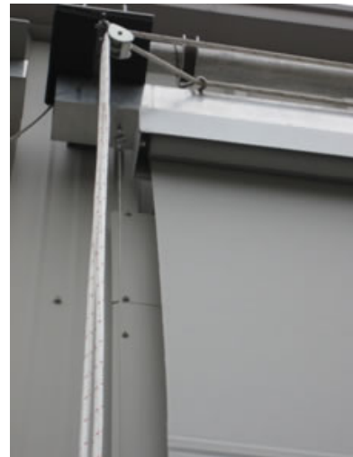
The lower hem bar is restrained by a vertical guide wire that runs the height of the window. Photo: LBNL.
