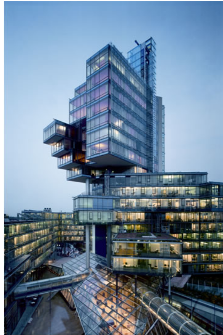
Nord/LB, Hannover, Germany, Behnisch Architekten Heliostats supplement daylighting at this building, but light is primarily provided through the generous glazing and transparent interior partition walls. Automated exterior venetian blinds manage both heat gain and glare. Photo: Roland Halbe
