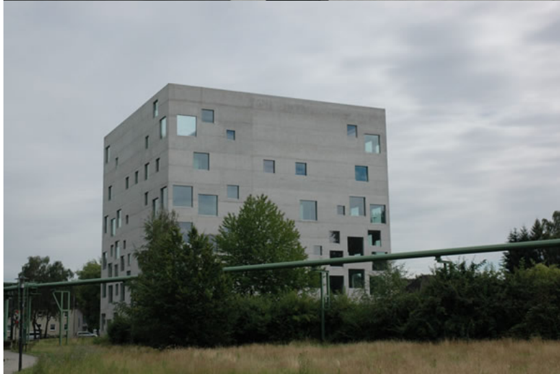
Zollverein School of Management and Design, Essen, Germany, SANAA Architect. Random but distributed window openings in the concrete building shell provide light and views with significantly reduced glazing area. Photo: Mark Perepelitza
