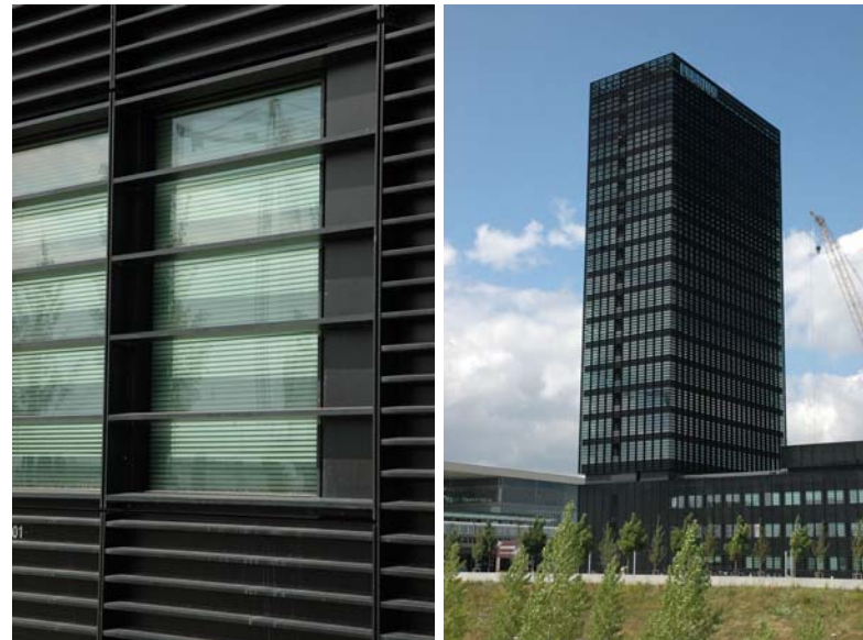
Copenhagen, Denmark, 3xn Architects. A uniform pattern of horizontal louvers provides sun shading but the dark color is not effective at redirecting daylighting. Photo: Mark Perepelitza
