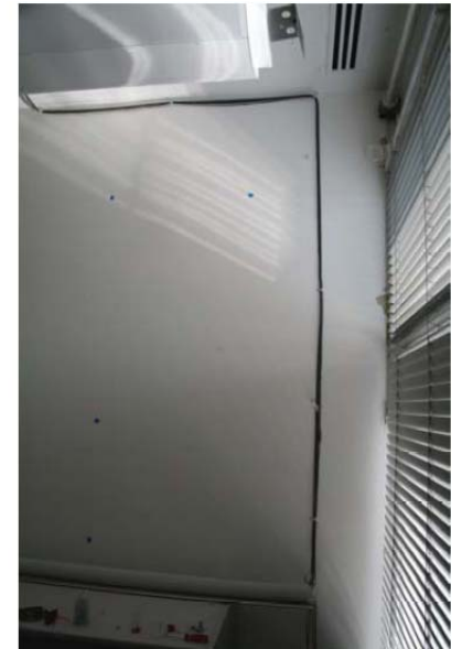
Automated sunlight-redirecting blind where the upper and lower slats are controlled simultaneously with a single header motor. The upper concave slats have a mirrored upper surface which reflects daylight towards the core of the building. Photos: LBNL.
