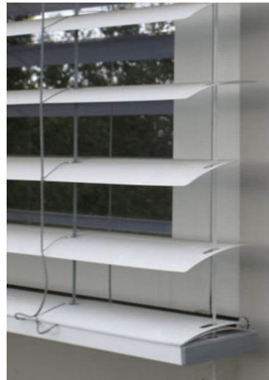
100-mm (3.9-inch) slats with semi-gloss white finish on top and bottom surfaces resting on braided plastic string ladders. Flat Trevira-polyester ribbons are used for lift function (above). Translucent Perlon cable at end of slats (below) tensioned at base using stainless steel clip. Photos: LBNL.
