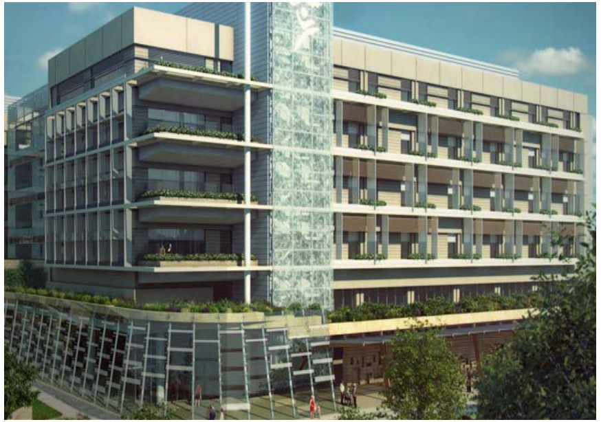
Rendering of highly externally shaded patient-wing of LPHC
