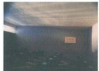
The light-redirecting light shelf (B) illuminates ceiling and upper wall surfaces, creating a brighter quality space for the same workplane illuminance level.
