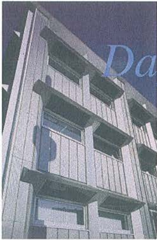
Daylighting system on a European building
